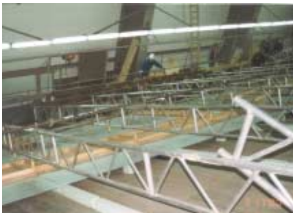
Insulation work on upper-sloped side.
