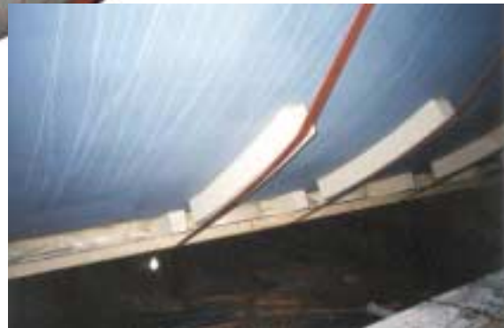
Insulation applied by moulding system on cylindrical tank
