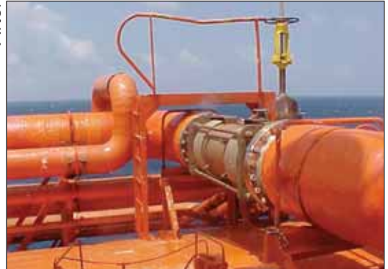
After maintenance and replacement of pipe insulation
