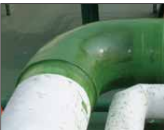
Prefabricated sections replacing defect bend insulation
